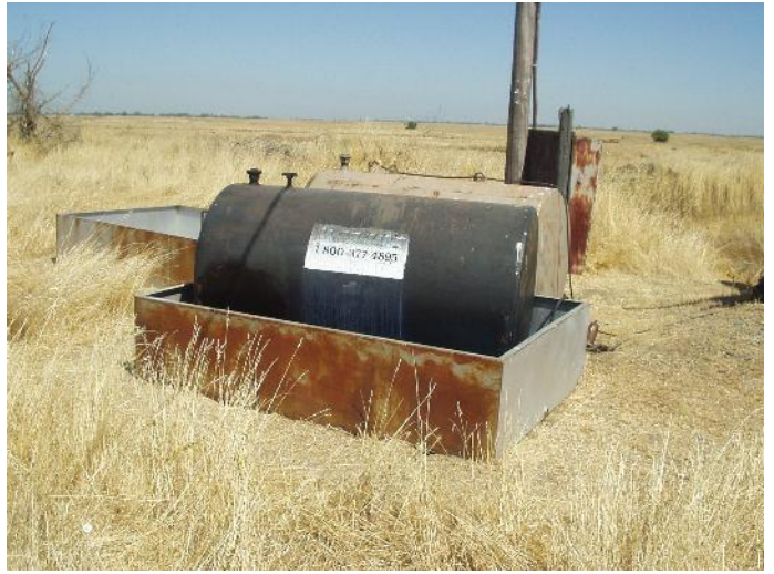
ABOVE GROUND FUEL TANKS ALONG SOUTHERN BOUNDARY OF PROPERTY VIEW TO NORTH
