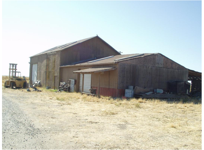
BARN-WORKSHOP LOCATED IN NORTHERN PORTION OF THE PROPERTY VIEW TO SOUTHEAST
