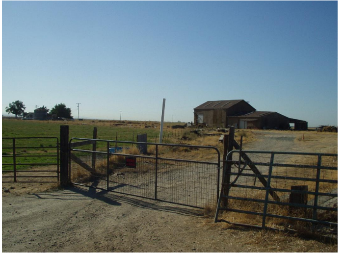
INTER SITE ENTRANCE VIEW TO SOUTHEAST
