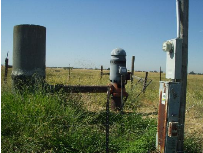
NORTHERN WELL VIEW TO SOUTH
