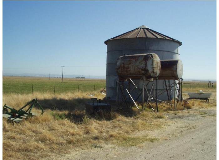
STEEL SILO AND ABOVE GROUND FUEL TANKS VIEW TO EAST
